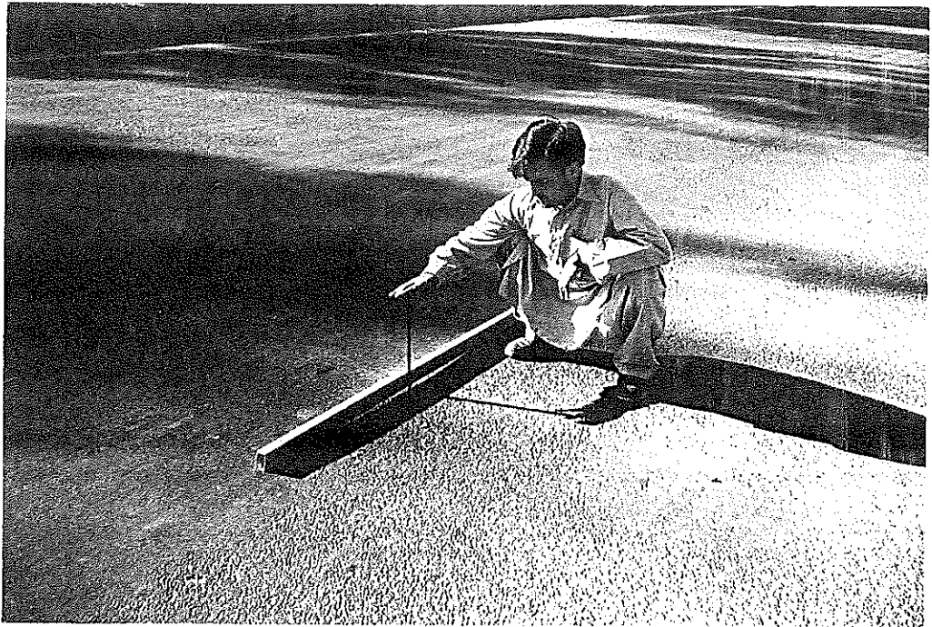
Plate 2 : SURFACE ROUGHNESS IS BEING CHECKED WITH STRAIGHT EDGE
